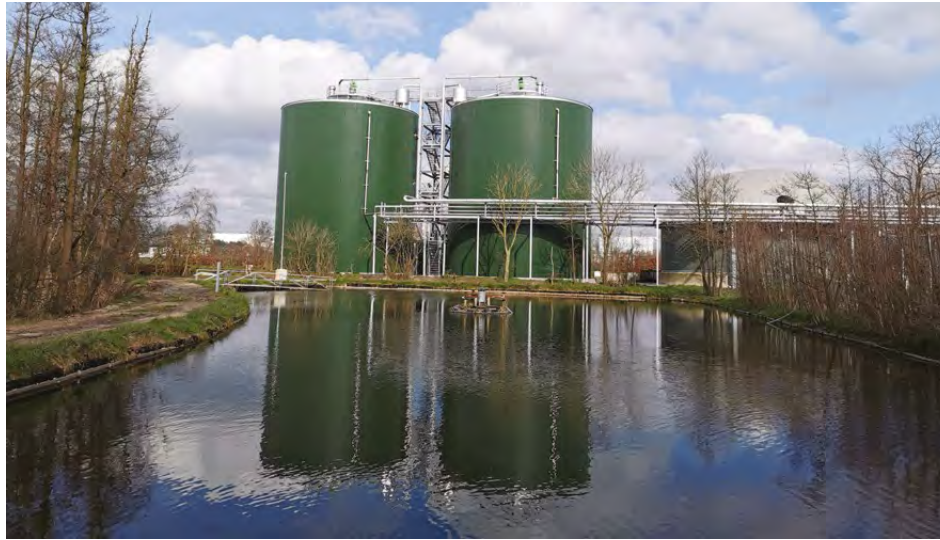
The digester in operation, fully wrapped in insulation and cladding.
