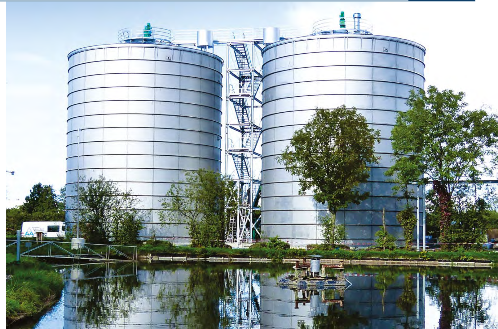
The CSTR's after installation, before insulation and cladding was installed.
