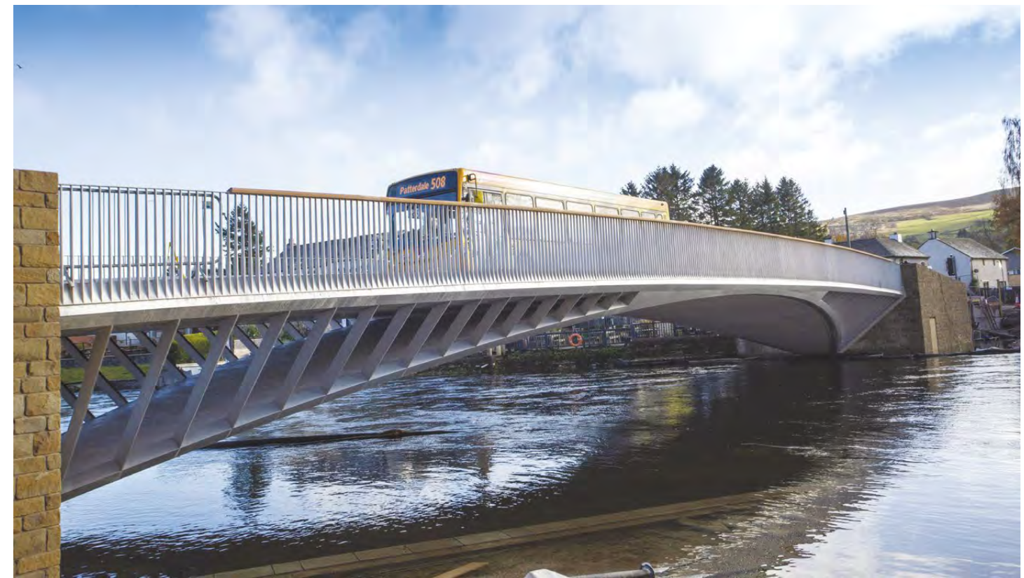
UK's first stainless steel road bridge was officially opened on Friday 23 October 2020 over the River Eamont at Pooley Bridge. It was designed by Knight Architects and uses duplex supplied by Outokumpu. Photo Courtesy of Outokumpu.
